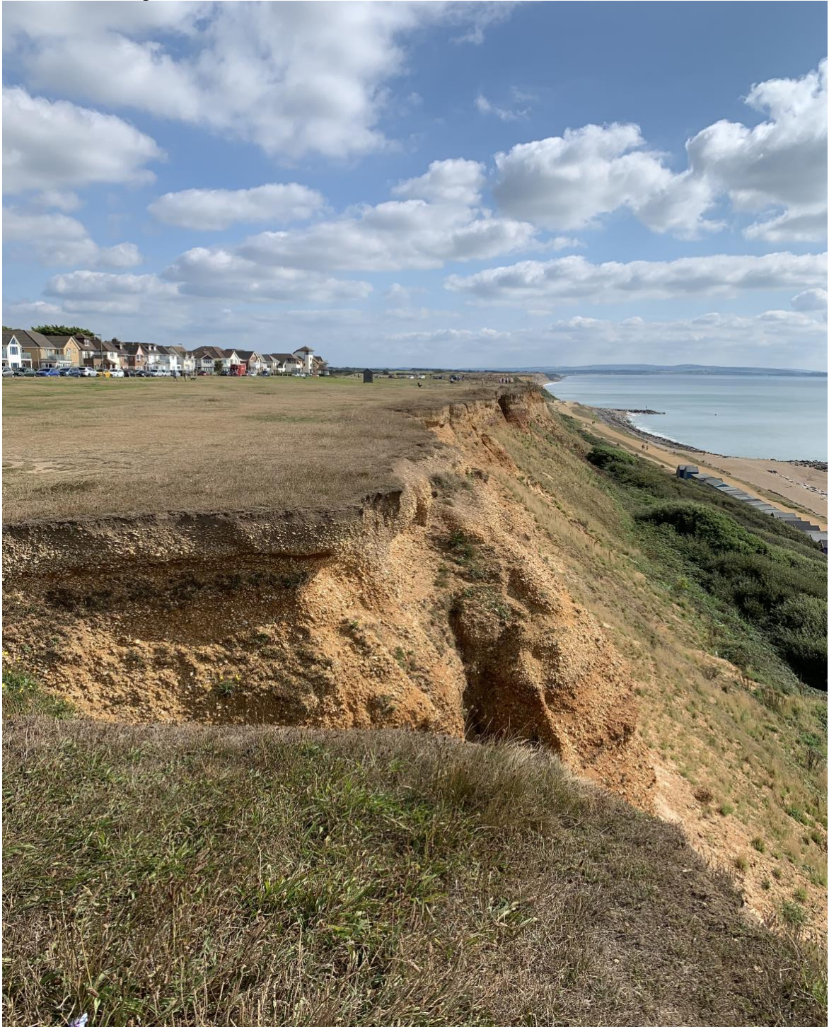
Photo 1 above shows how erosion has undercut the cliff edge causing an overhang in places.
